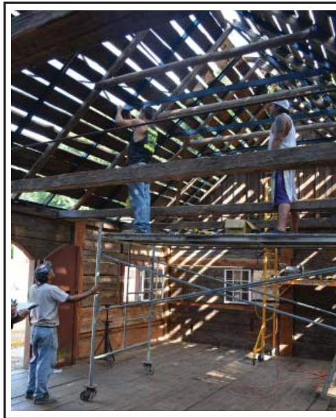
Granary repairs completed 2013!
